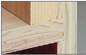
The bottom fits into a dado cut in the carcass side. The toe kick supports the bottom.
