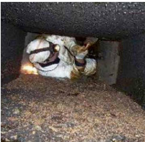
Figure 19: Checking and cleaning ductwork.
