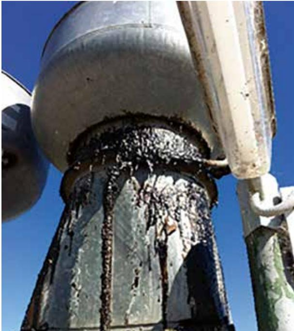
Figure 15: Grease leaking from ducts and pooling on roof.
