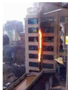
**Figure 18: Fire rapidly spreading up a vertical kitchen exhaust duct.**
